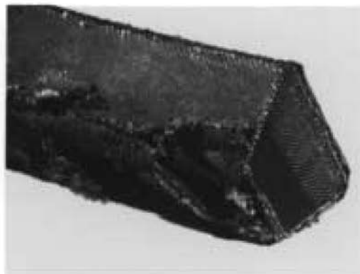
Cover Fabric Rupture
