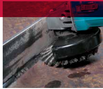
Cleaning a fillet weld with a bevel brush.
