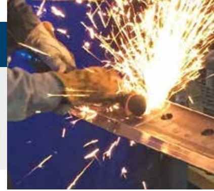
Type 18R plug used to grind I.D. bevels and flatten surface on rail frog section.
