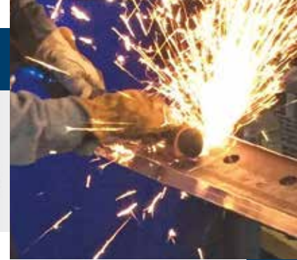
Type 18R plug used to grind I.D. bevels and flatten surface on rail frog section.
