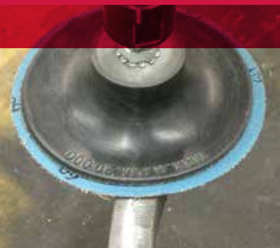
Blending surface imperfections prior to painting.
