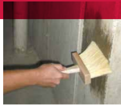
Applying waterproofing material with a masonry brush.
